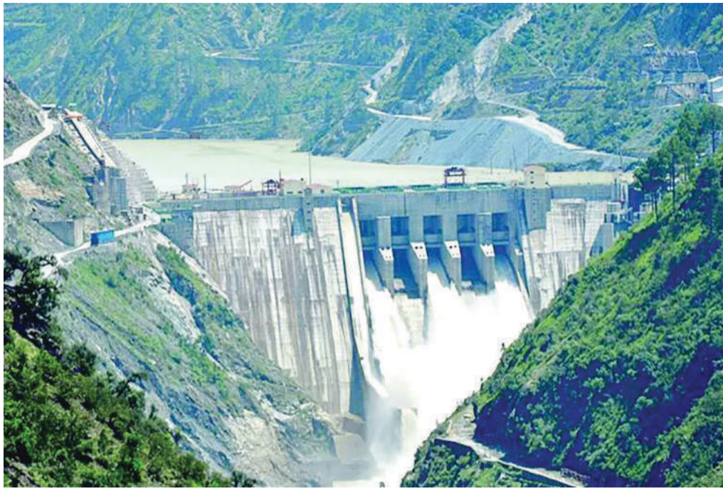
assessed for feasibility and cost. The remarks come amid wider discussions on strengthening India's power infrastructure to keep electricity supply ahead of rising demand.
