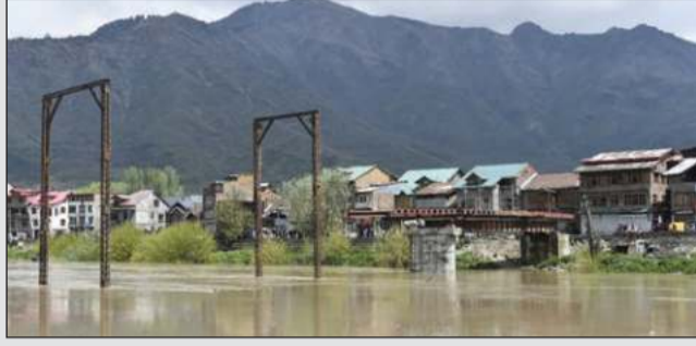
of over 15 crucial bridges and around 07 footbridges in the Kashmir valley remains unfinished, despite commencing
