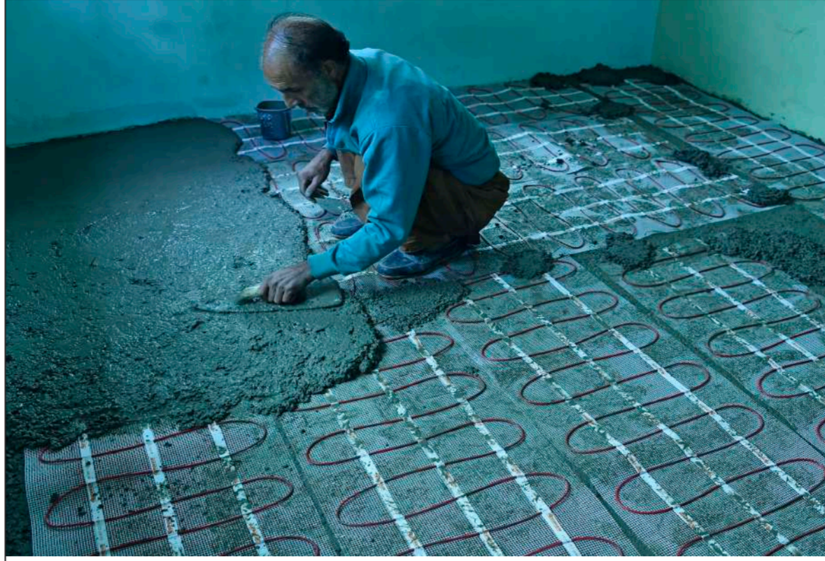
As cold conditions intensified across Kashmir, demand for underfloor heating system picks up amid worsening power crises. KO Photo, Abid Bhat
