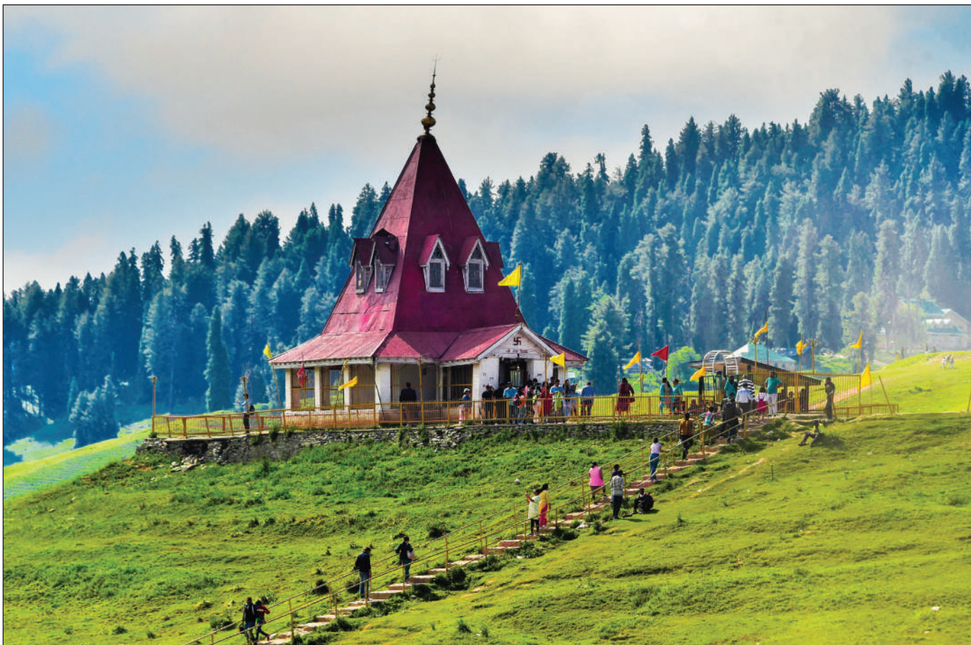
SHIV TEMPLE CONSTRUCTED IN 1915 during Maharaja Hari Singh's rule is a major attraction for tourists in the picturesque meadow of Gulmarg in Baramulla: KO Photo, Abid Bhat
