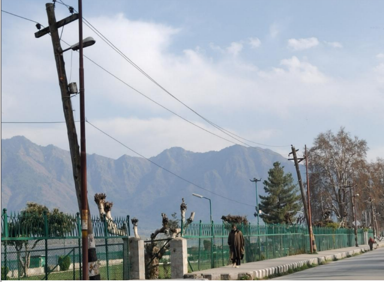
POLES APART: Despite erecting new electric poles, the old poles are still standing their ground in Hazratbal, Srinagar.
